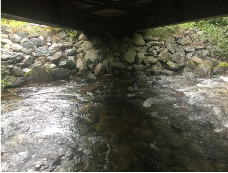
Left Bank Abutment when facing downstream
