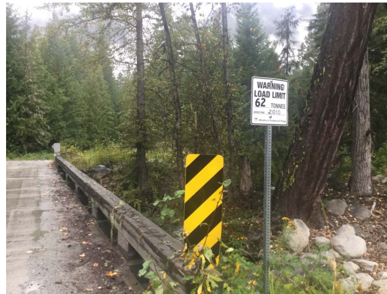
Load Rating Sign
